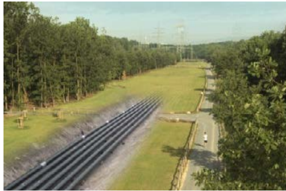
Figure 1.2 left side: view into a tunnel with two GIL systems and elastic bending, Paulaner Munich; right side: directly buried GIL at Kelsterbach, close to Frankfurt Airport
