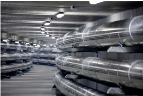
Figure 1.2 left side: view into a tunnel with two GIL systems and elastic bending, Paulaner Munich; right side: directly buried GIL at Kelsterbach, close to Frankfurt Airport
